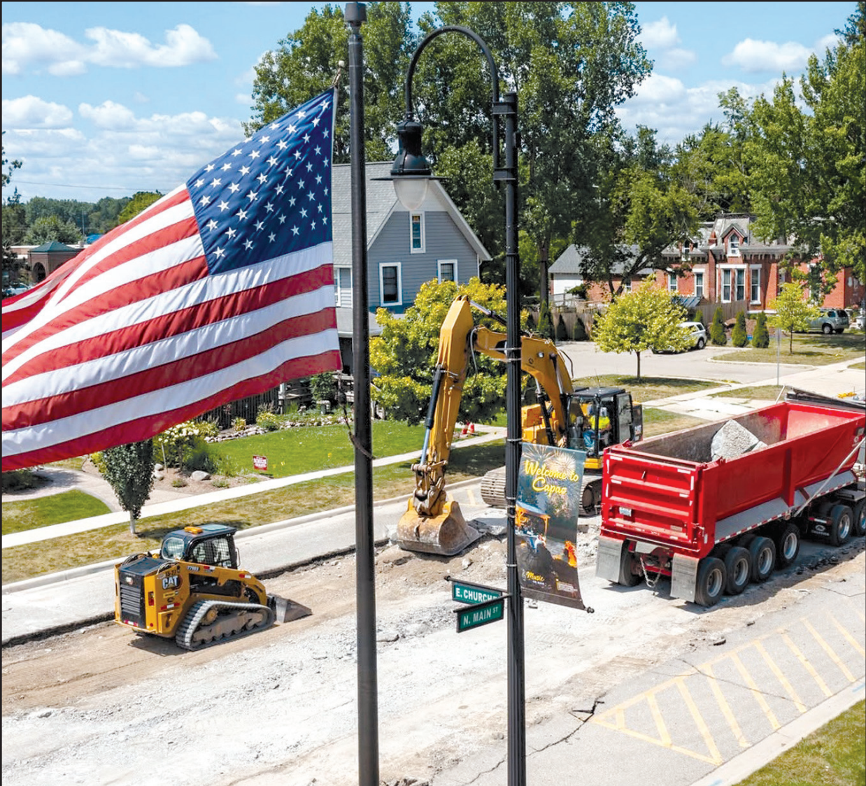
With barricades in place throughout town in Capac, crews work to remove the roadway last week.
