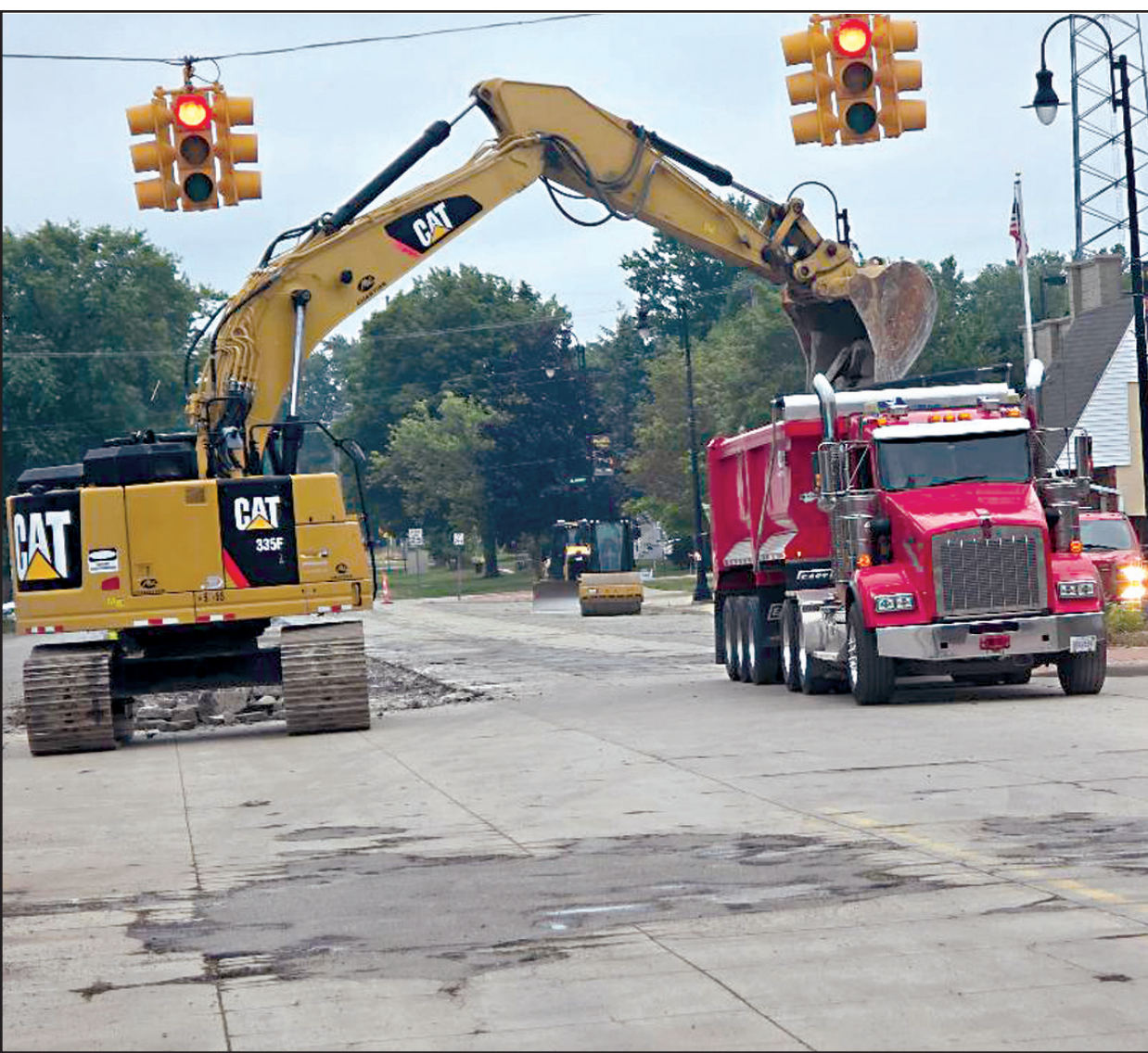
Heavy Equipment and large trucks were working on removing the old, decaying Main St. in Capac Tuesday morning.
