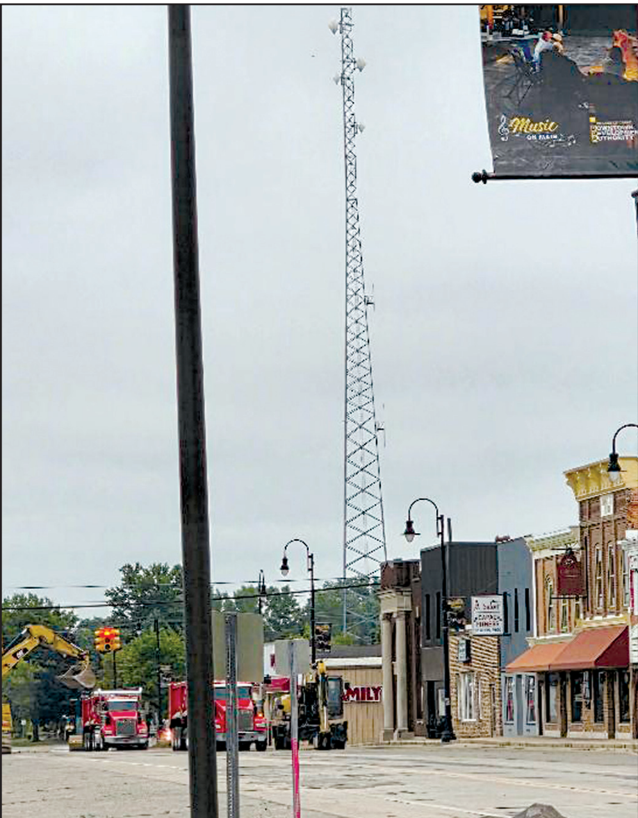
Downtown businesses will remain open during construction.
