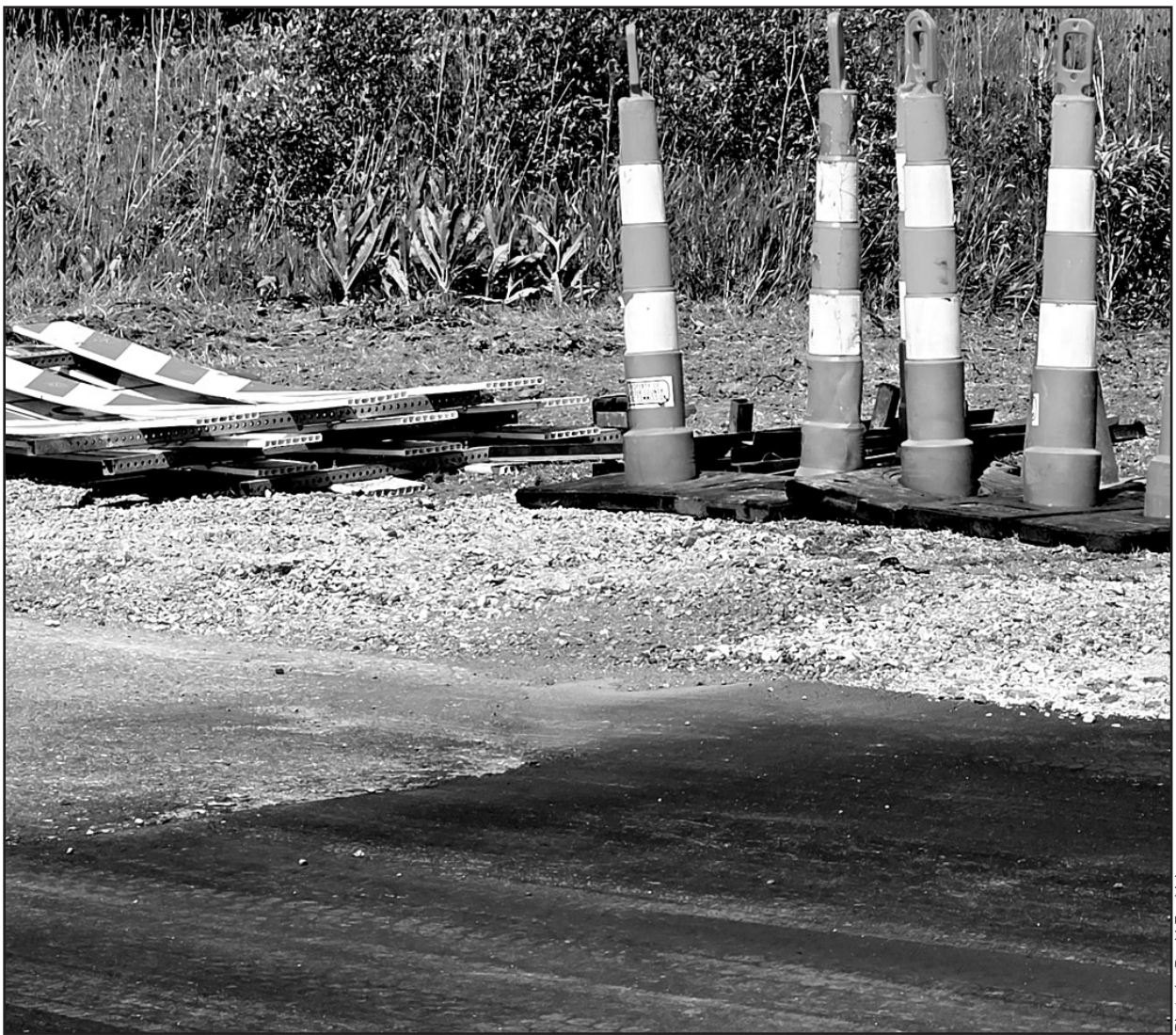
A small portion of Graham Rd. where a large culvert was installed, was paved following construction by the Lapeer County Road Commission. The road was opened last week before the 4th of July holiday.
